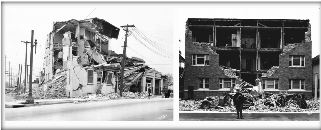
Figure 1. Collapse of unreinforced masonry building, California 1933
