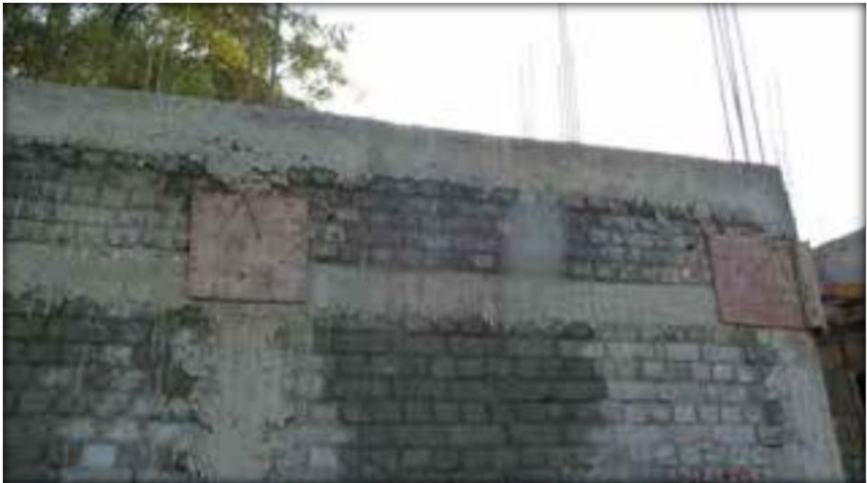
Figure 30. Masonry and RC-tie-column construction above the lintel band level
