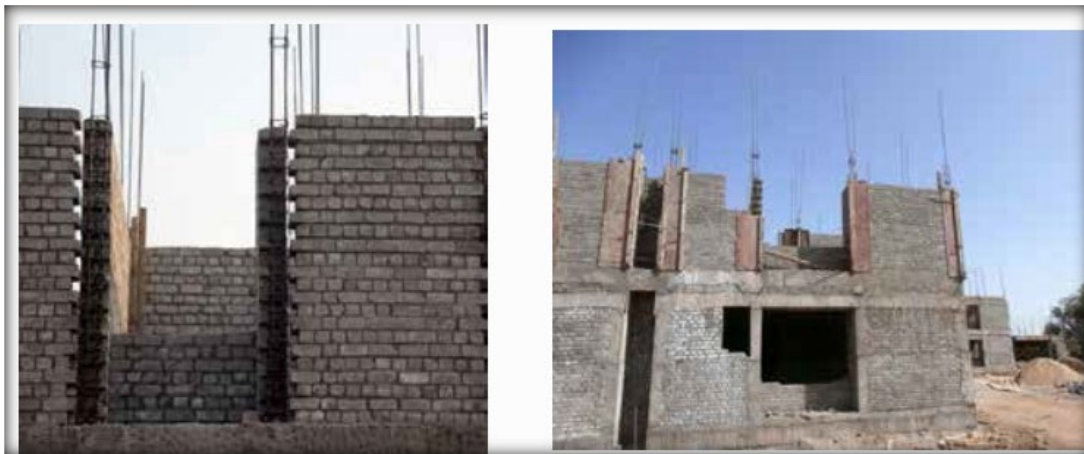
Figure 34. Anchorage of Longitudinal Bars: T-connection
