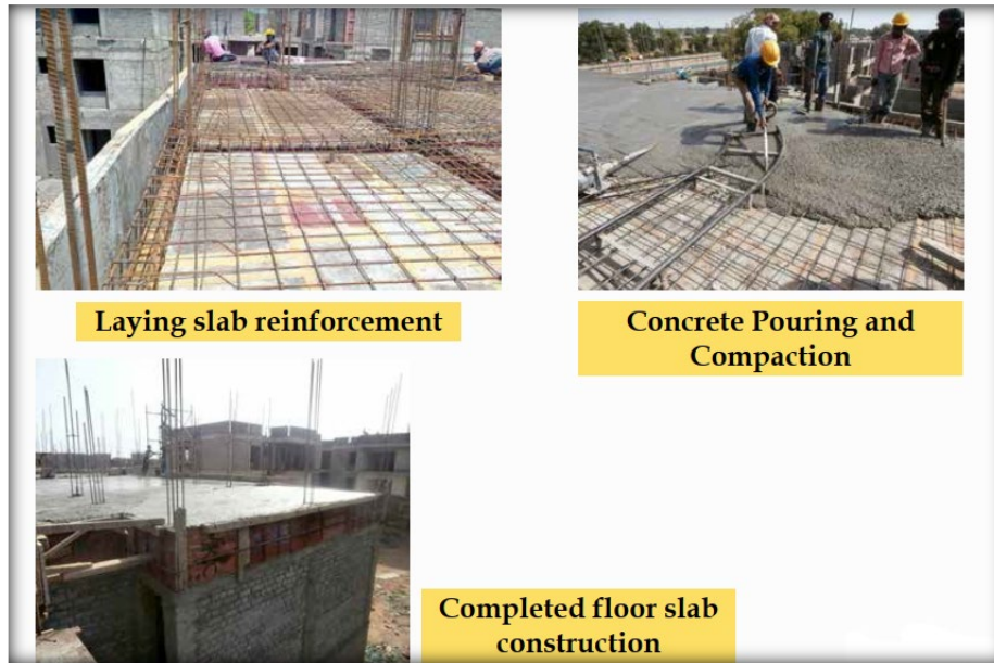
Figure 38. Construction of Slab
