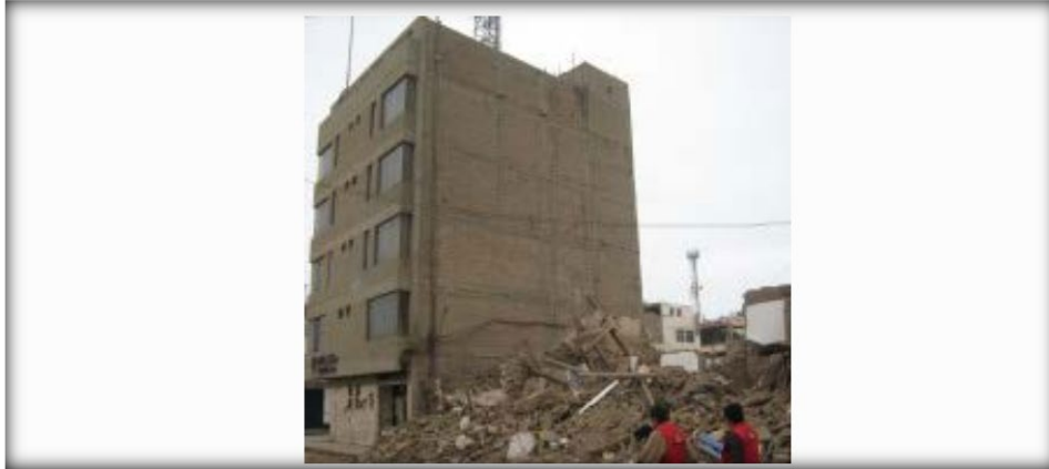
Figure 4. Confined masonry building in M8.0 2007 Pisco, Peru Eqk (Collapse of nearby adobe house)
