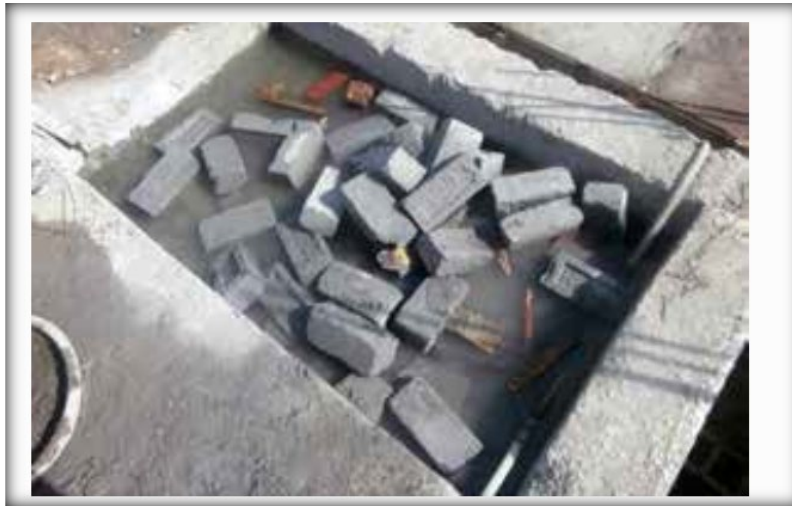
Figure 23. Bricks immersed in water before construction
