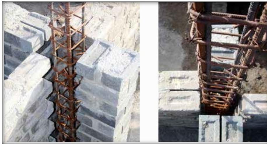
Figure 27. Tothing at cross wall intersections
