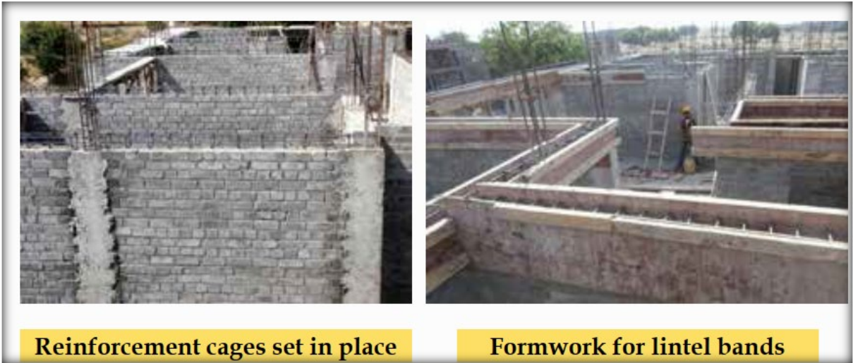
Figure 29. Construction of RC lintel bands
